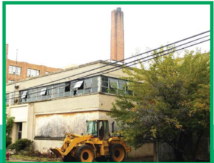
The former automotive site before cleanup and demolition activities.
