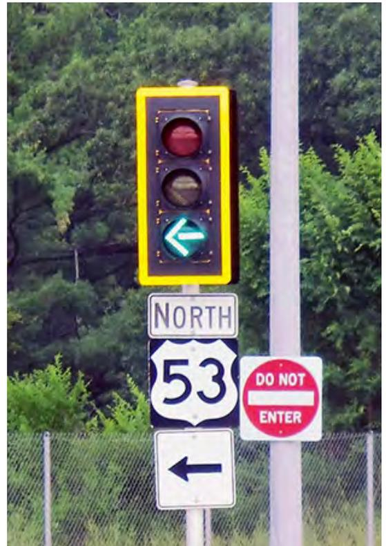
Example of a signal backplate framed with a retroreflective border.
