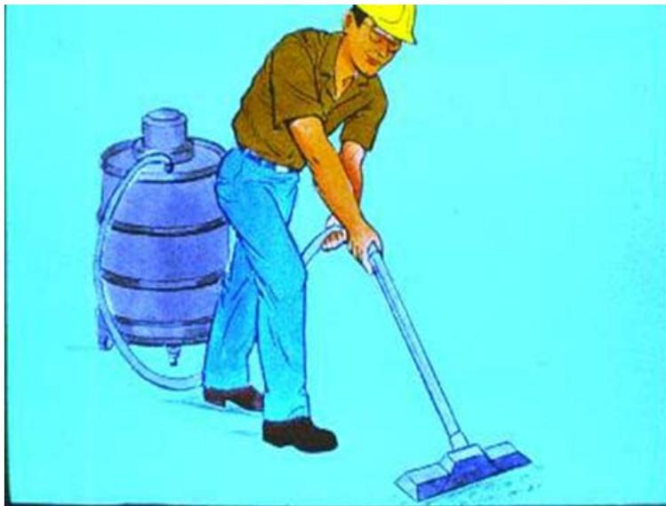
**Figure 64.** Using a vacuum system to collect dust
