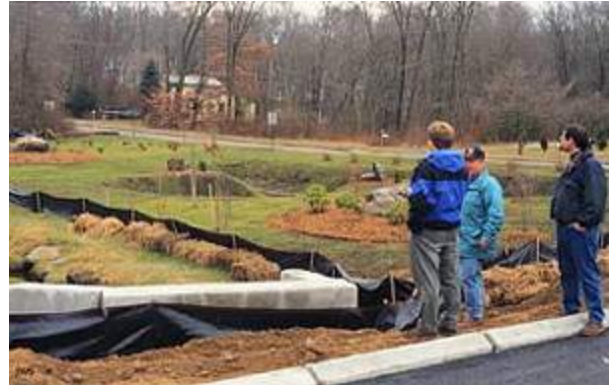
Construction reviewers periodically inspect construction sites to ensure that contractors have installed and maintained their erosion and sediment controls properly (Source: University of Connecticut Cooperative Extension System, 2000)
