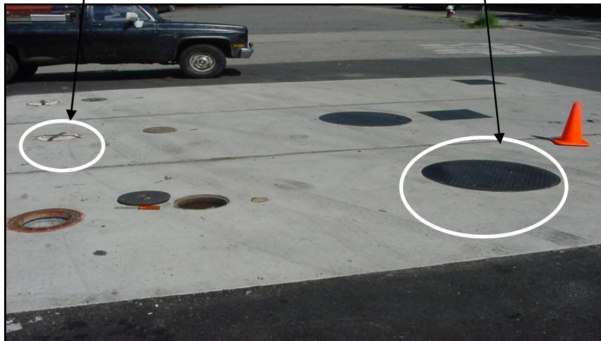
View of sump lids
