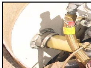
Sump penetration seals in good condition
