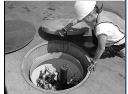
Person wearing safety gear while inspecting a sump
