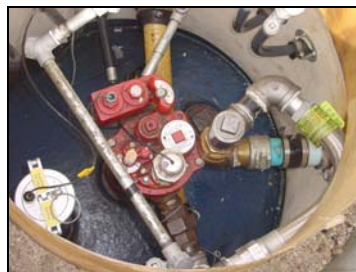
Contained turbine sumps and equipment in good condition
