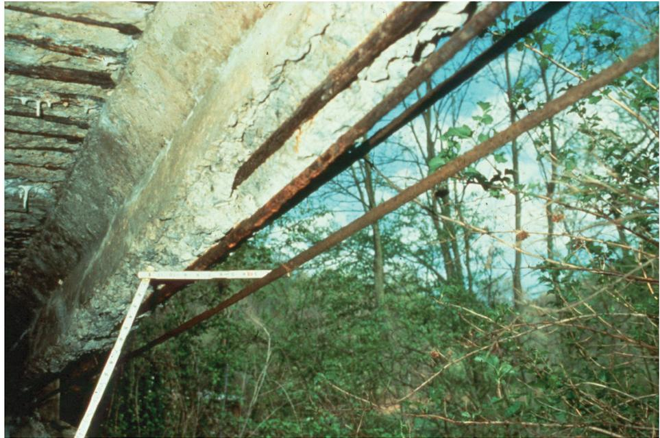
**Figure 2.2.26** Loss of Bond: Concrete / Corroded Reinforcing Bar
