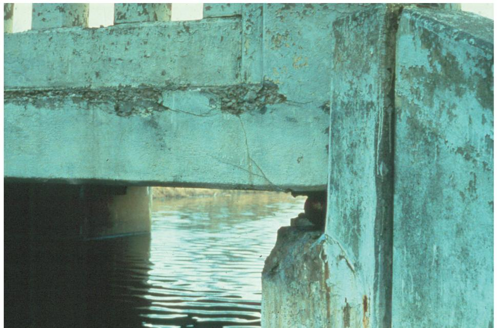
**Figure 2.2.8** Shear Crack on a Slab Beam
