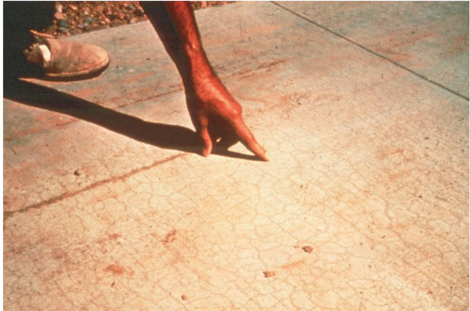
**Figure 2.2.15** Pattern or Map Cracks
