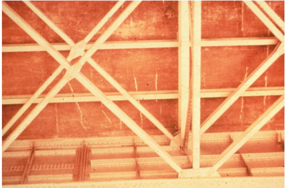
**Figure 2.2.13** Transverse Cracks
