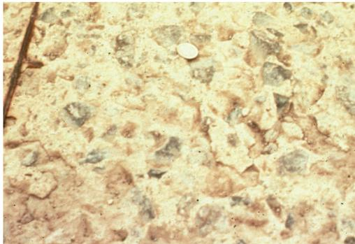
**Figure 2.2.19** Severe Scaling
