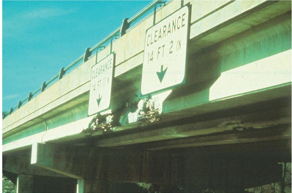
**Figure 2.2.24** Collision Damage to Prestressed Concrete I-Beam
