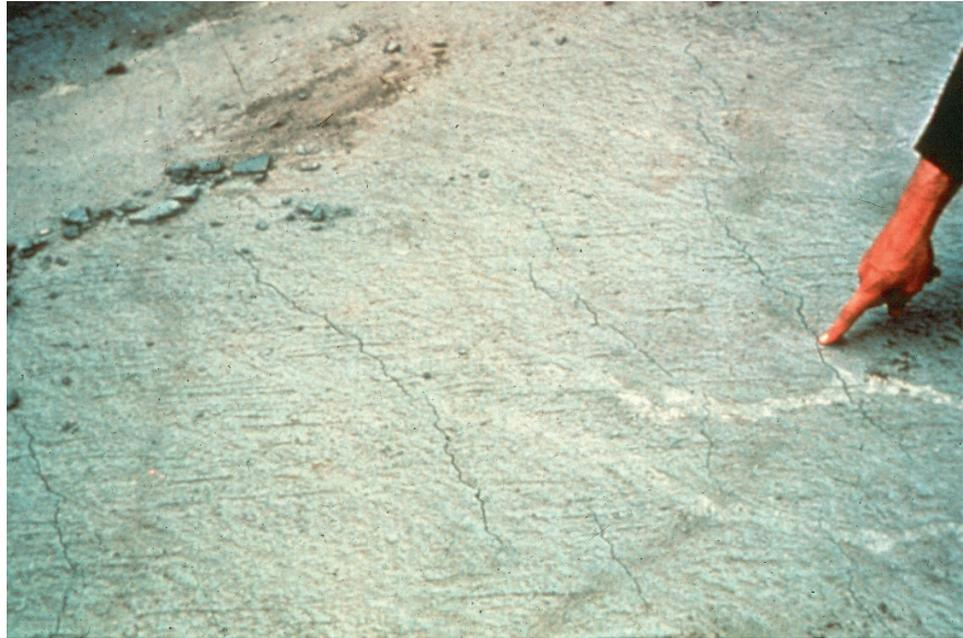
**Figure 2.2.11** Temperature Cracks
