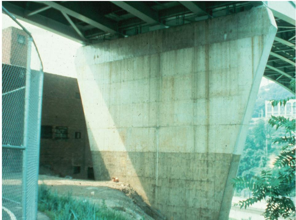
**Figure 2.2.28** Anti-Graffiti Coating on Lower Area of Bridge Piers
