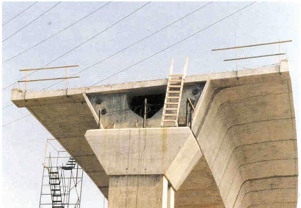
**Figure 2.2.5** Post-tensioned Concrete Box Girder
