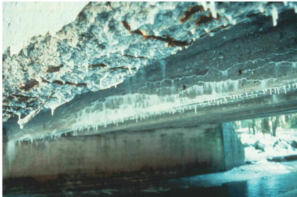
**Figure 2.2.21** Efflorescence
