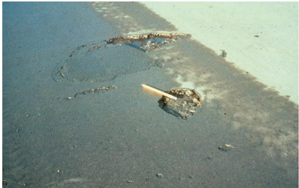
**Figure 2.2.20** Spalling on a Concrete Deck
