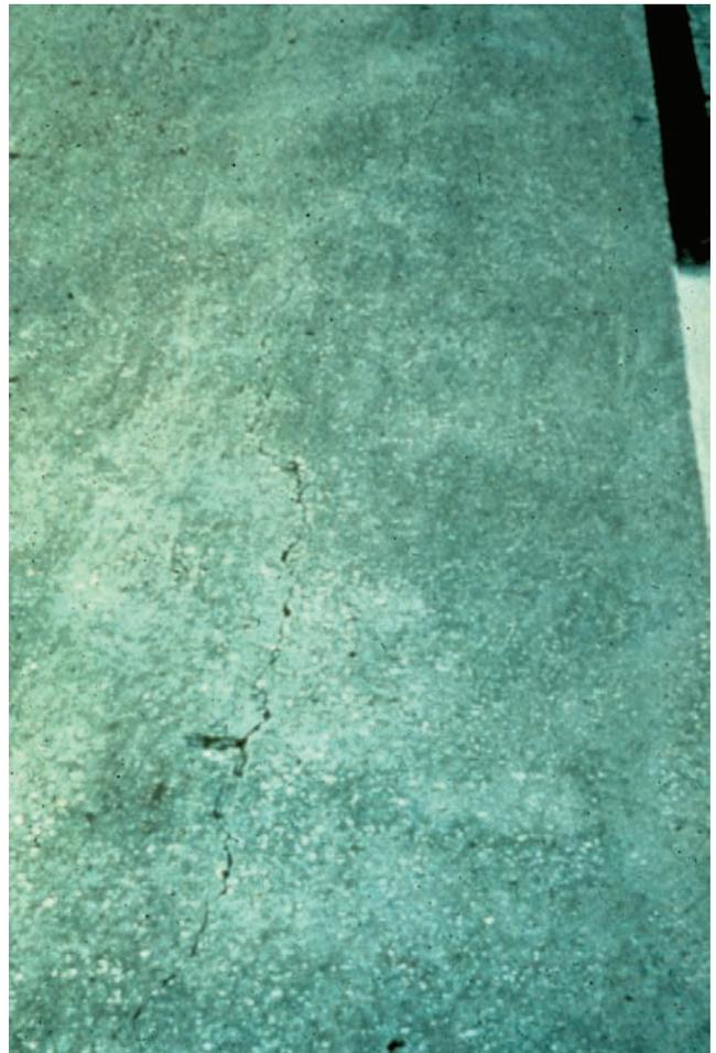
**Figure 2.2.14** Longitudinal Cracks
