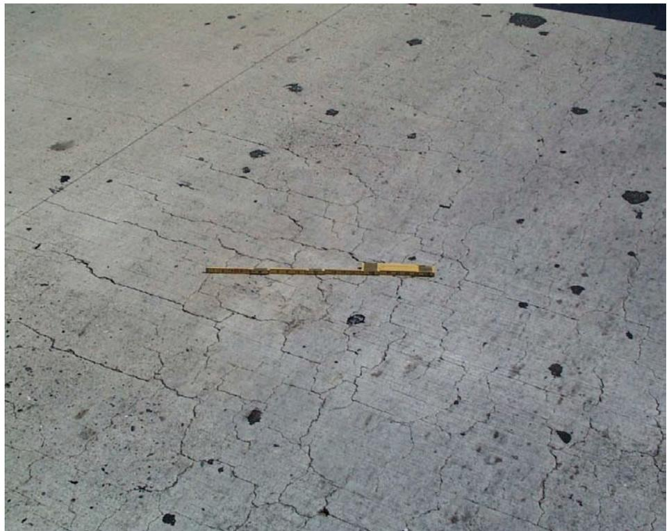
**Figure 2.2.12** Shrinkage Cracks
