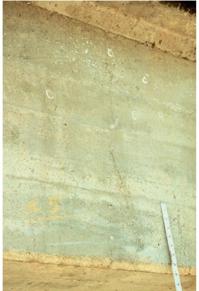
**Figure 2.2.7** Flexural Crack on a Tee Beam
