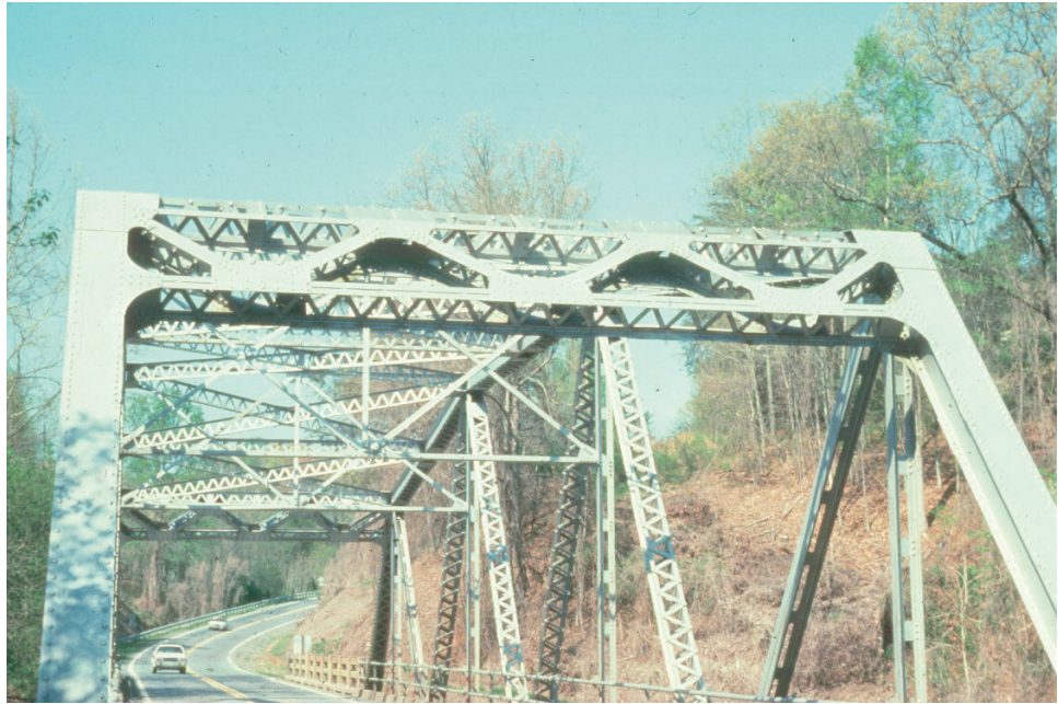
Figure 8.6.40 Portal Bracing
