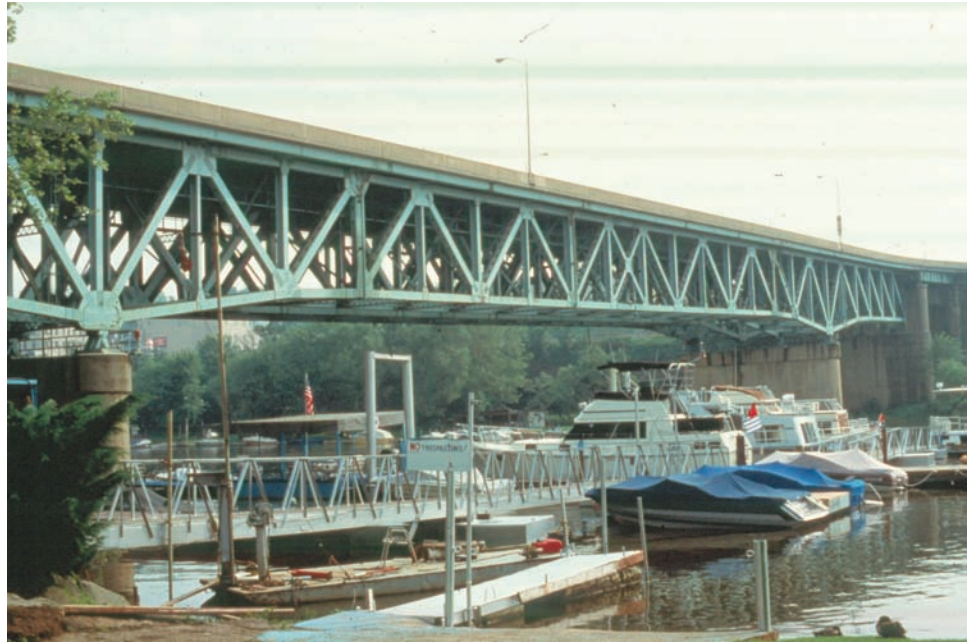
Figure 8.6.16 Cantilever Deck Truss
