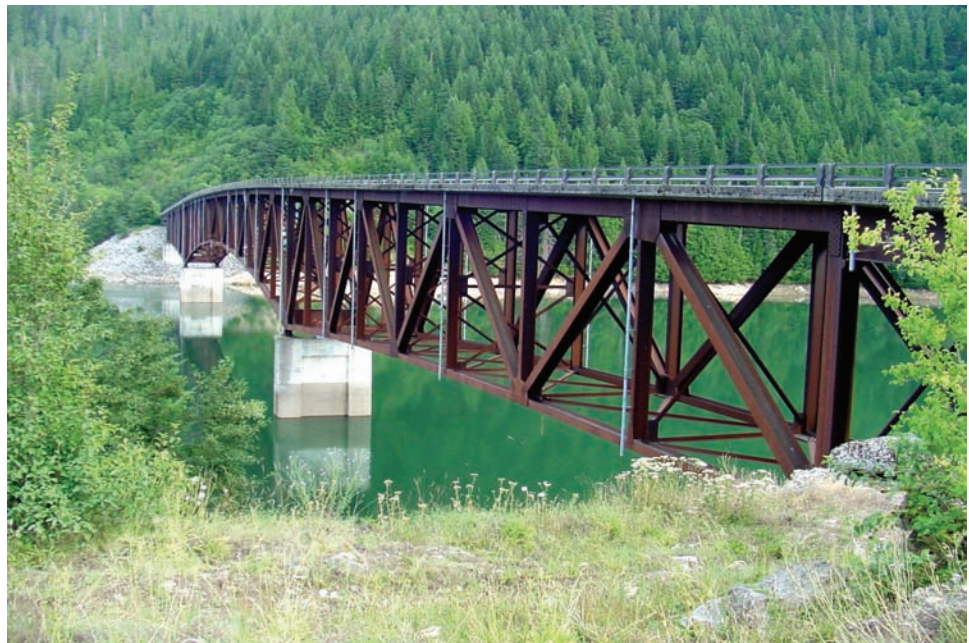
Figure 8.6.5 Deck Truss
