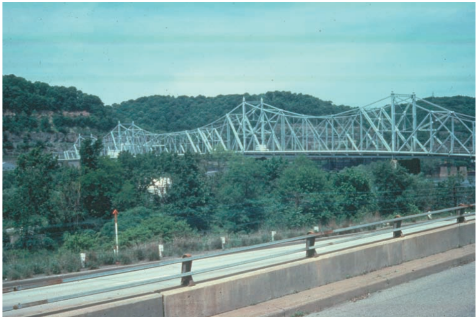
Figure 8.6.15 Cantilever Through Truss
