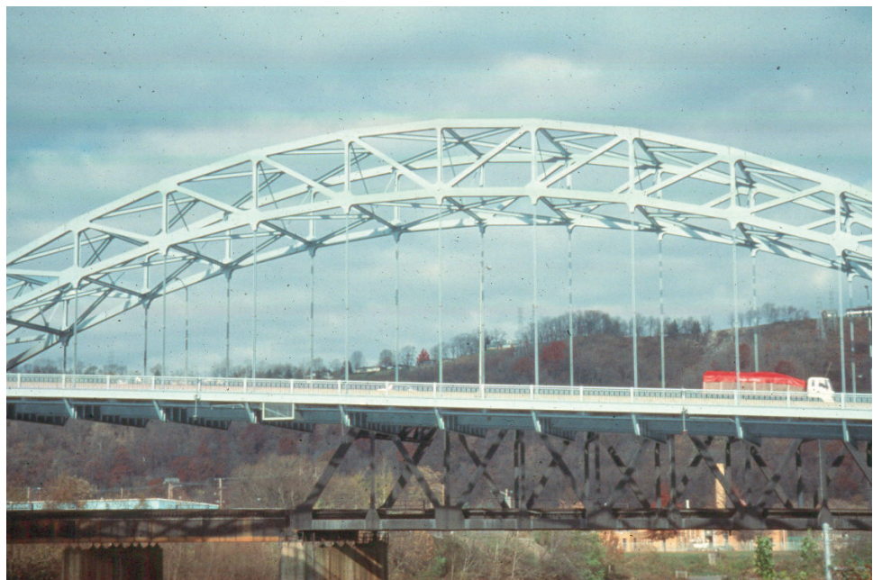
Figure 8.6.7 Arch Bridge with Stiffening Truss
