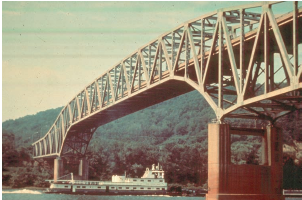
Figure 8.6.3 Through Truss
