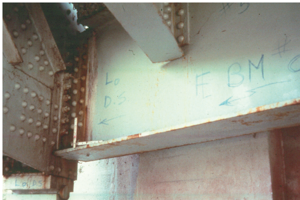
Figure 8.6.59 Clip Angles at Floorbeam and Stringer Connections
