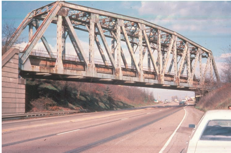
Figure 8.6.22 Single Span Through Truss – General Elevation View
