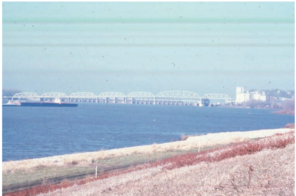
Figure 8.6.13 Multiple Span Through Truss
