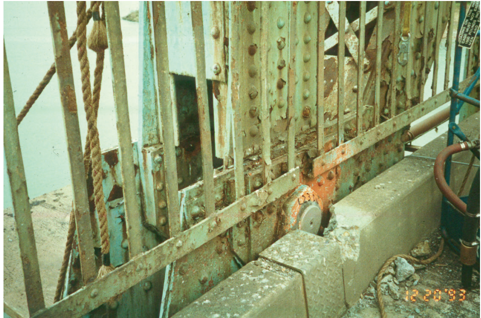
Figure 8.6.60 Suspended Span Pin
