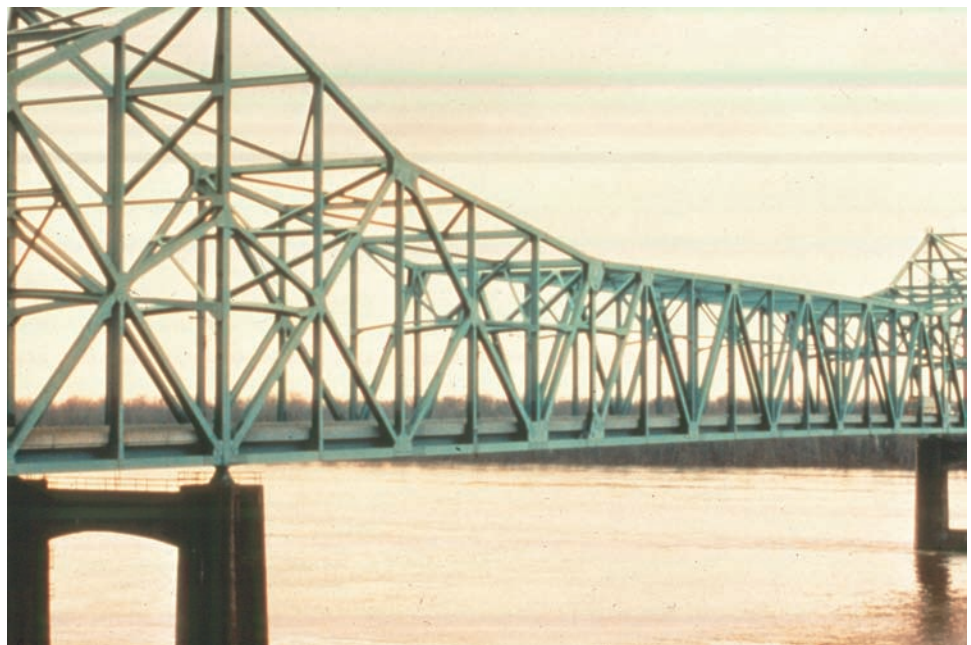
Figure 8.6.17 Cantilever Through Truss
