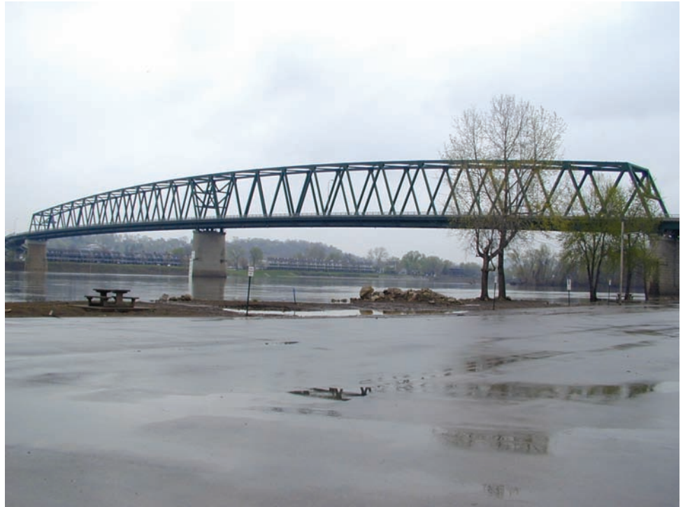
Figure 8.6.23 Continuous Through Truss
