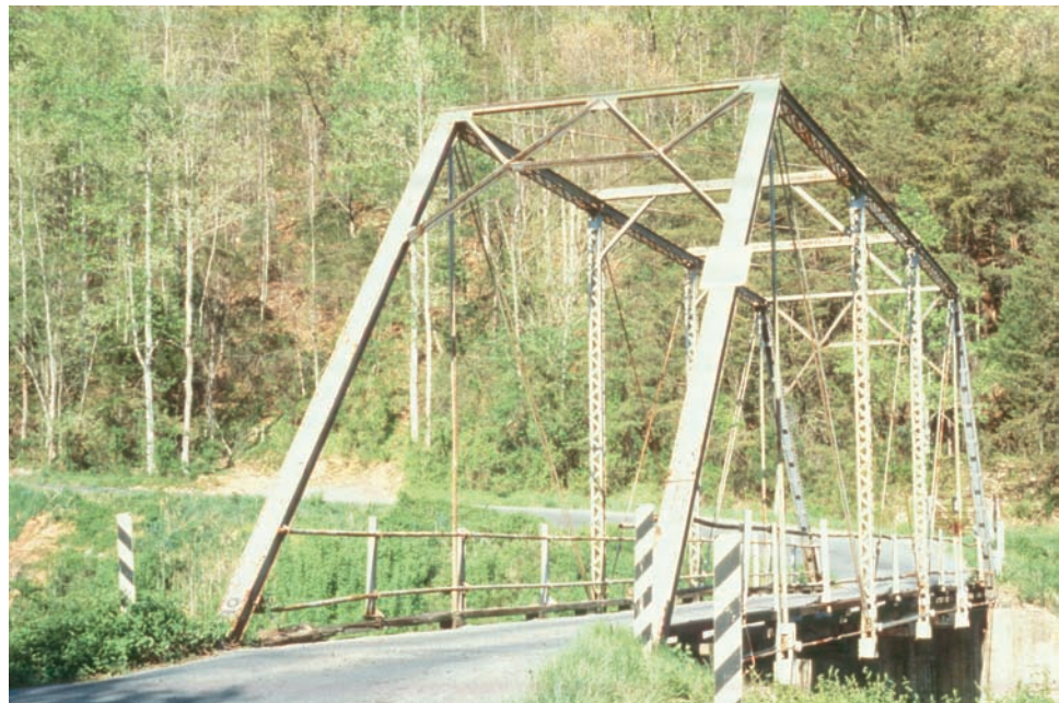
Figure 8.6.11 Single Span Through Truss
