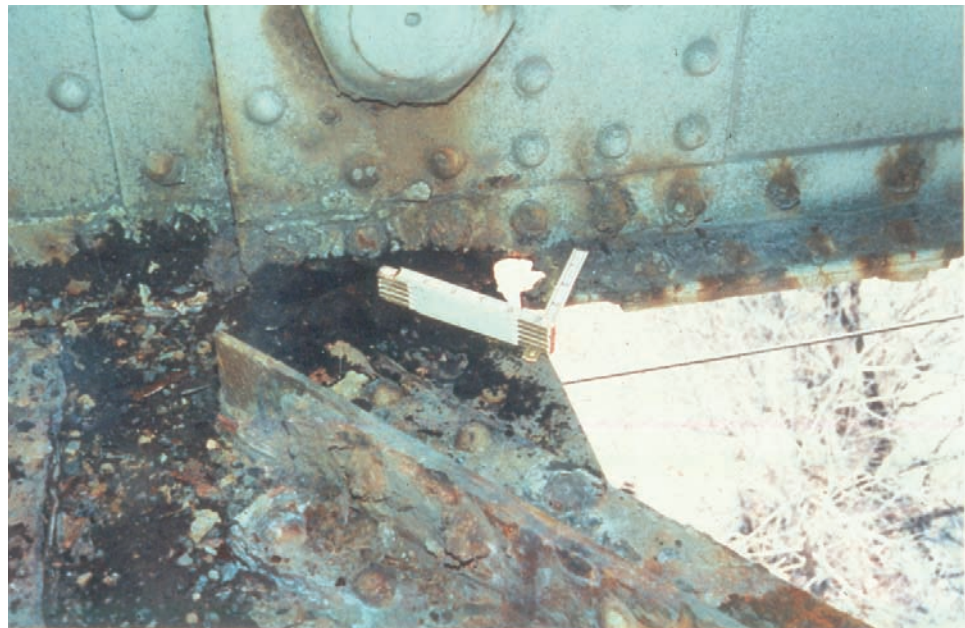
Figure 8.6.37 Lateral Bracing Gusset Plate and Lateral Bracing
