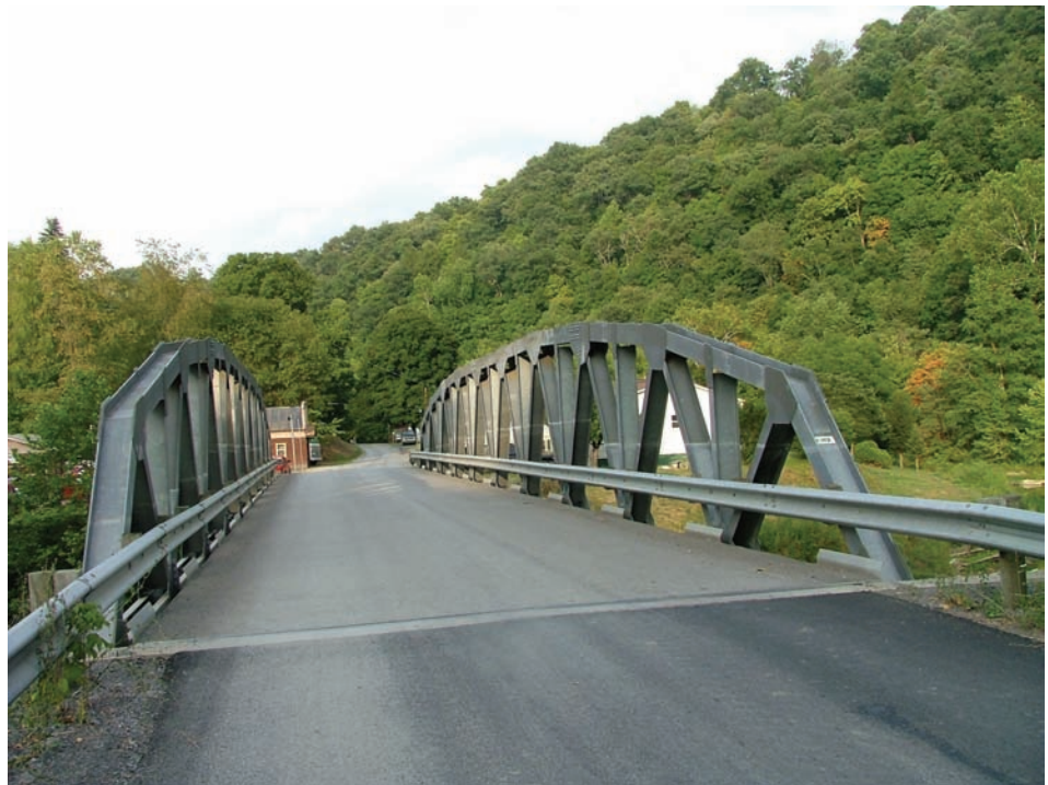
Figure 8.6.1 Single Span Truss
