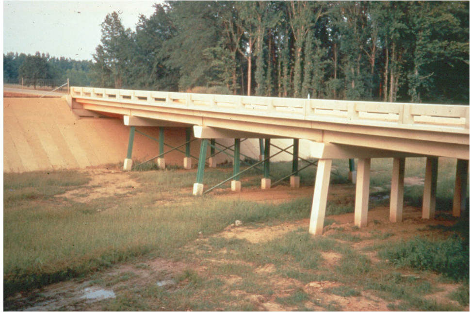
Figure P.1.76 Pile Bent
