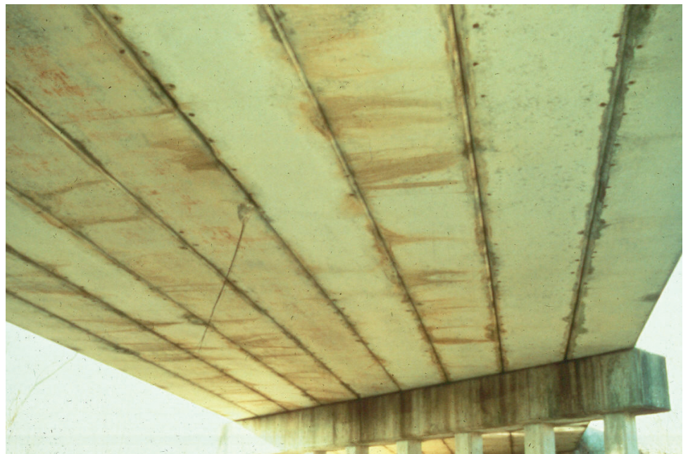
Figure P.1.51 Adjacent Box Beam Bridge
