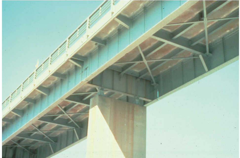
Figure P.1.48 Girder Floorbeam Stringer Bridge
