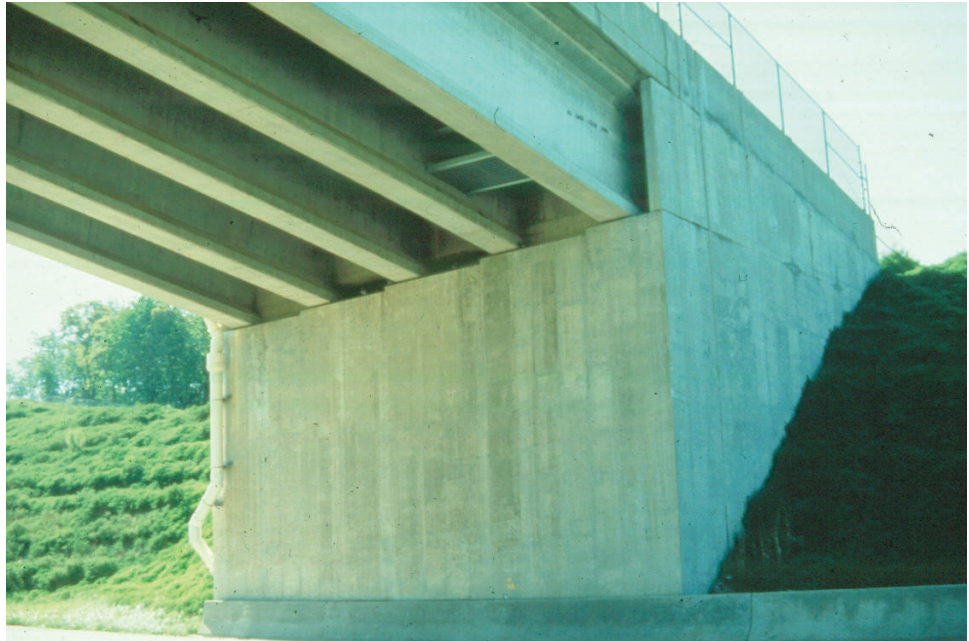
Figure P.1.65 Concrete Abutment
