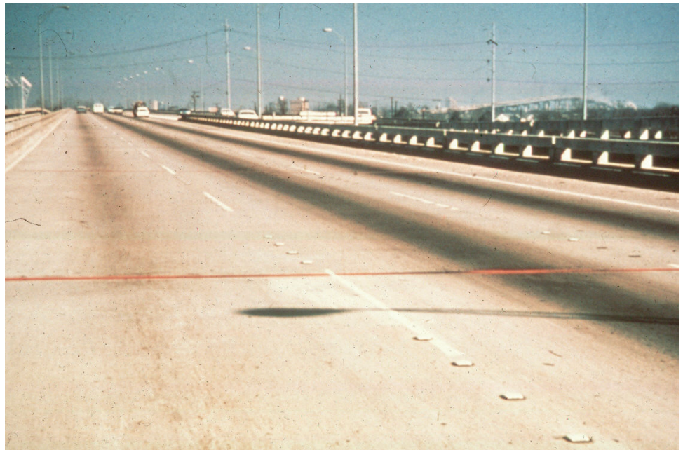
Figure P.1.24 Bridge Deck with a Smooth Riding Surface
