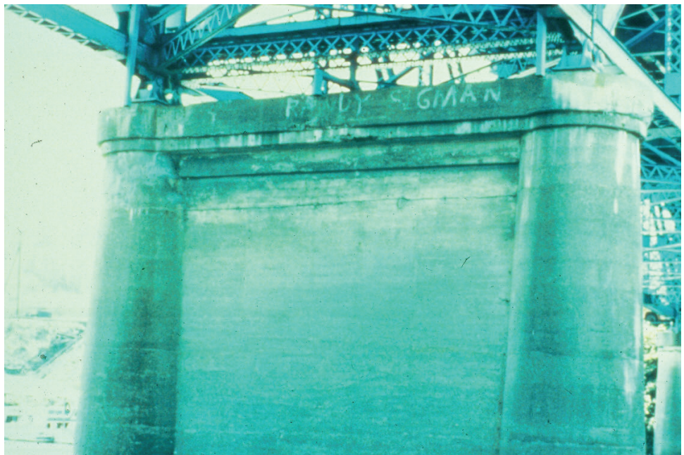
Figure P.1.73 Column Pier with Web Wall
