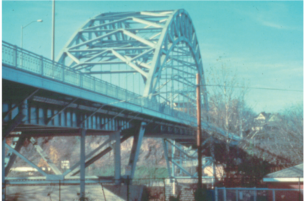
Figure P.1.56 Through Arch Bridge
