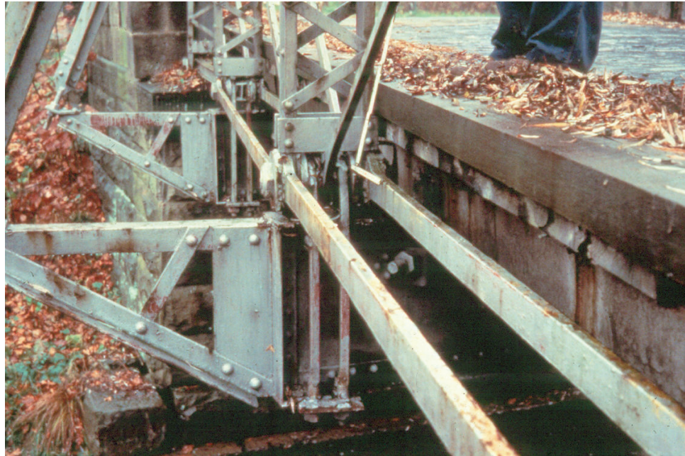
Figure P.1.18 Pin-Connected Truss Members
