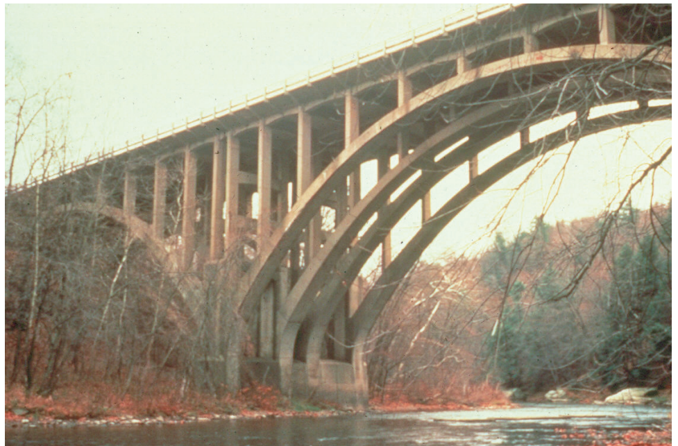
Figure P.1.55 Concrete Deck Arch Bridge
