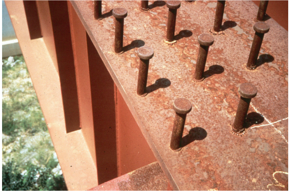
Figure P.1.27 Shear Studs on Top Flange of Girder (before Concrete Deck is Placed)
