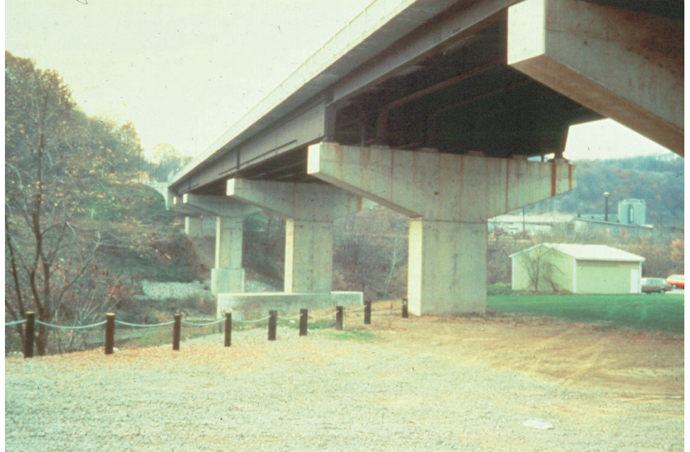
Figure P.1.74 Cantilever or Hammerhead Pier
