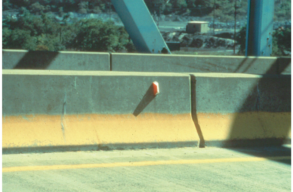
Figure P.1.36 New Jersey Barrier
