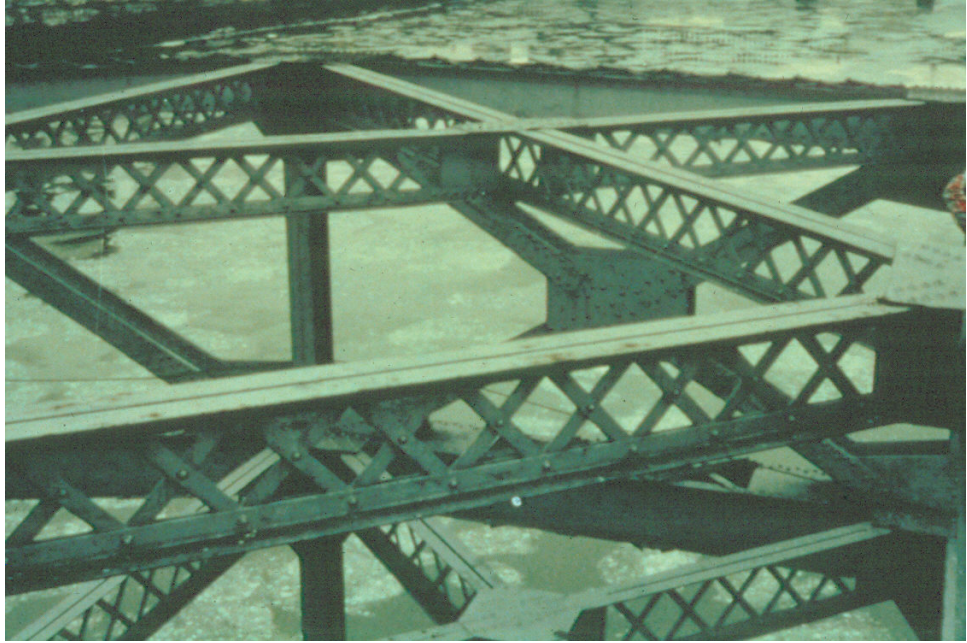
Figure P.1.11 Bracing Members Made from Angles, Bars, and Plates
