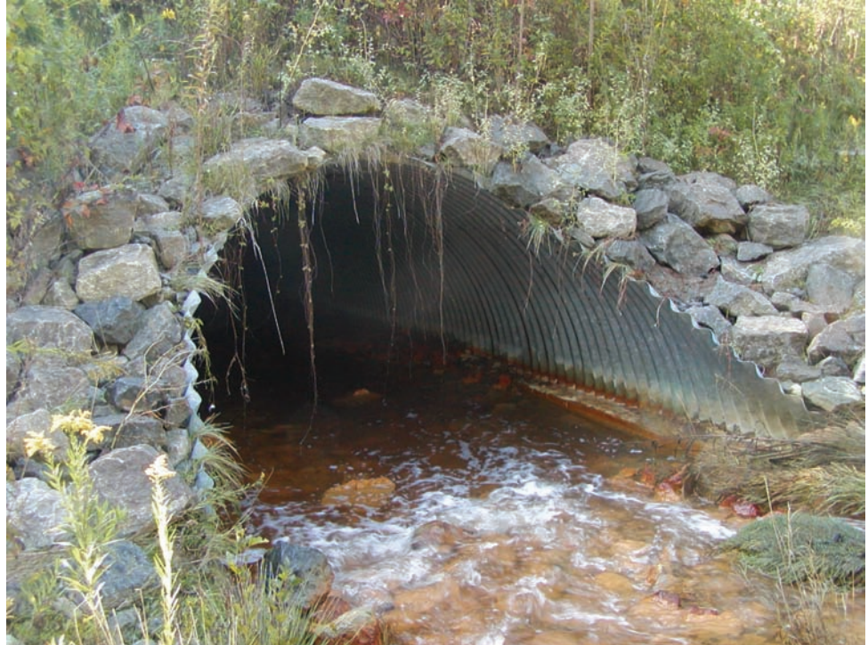
Figure P.1.63 Culvert
