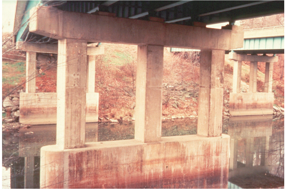
Figure P.1.66 Concrete Pier
