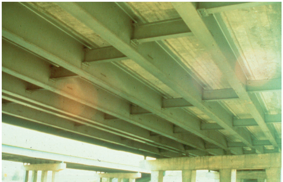
Figure P.1.41 Diaphragms
