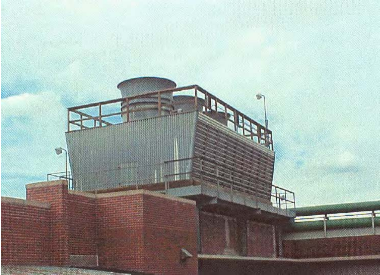
Figure 7 Cross-Flow Cooling Tower
