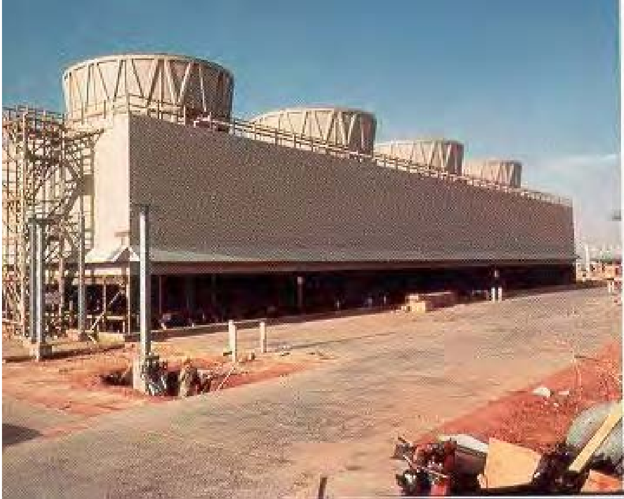
Figure 9 Counter-Flow Cooling Tower
