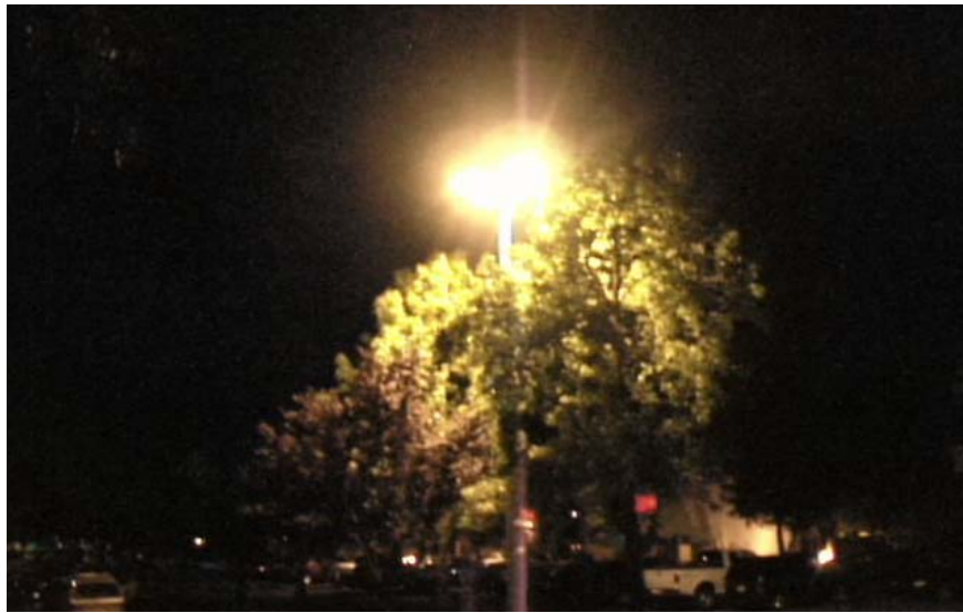
Figure 2 (continued) Examples of direct glare
