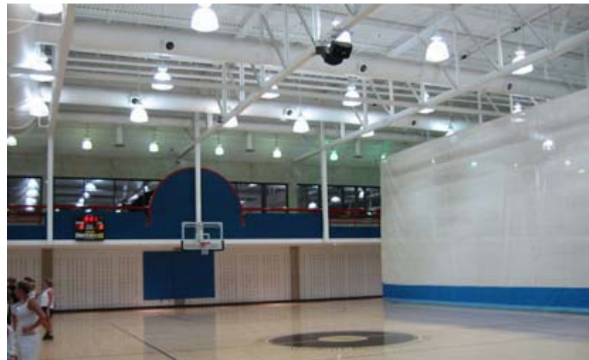
Figure 2 Examples of direct glare
