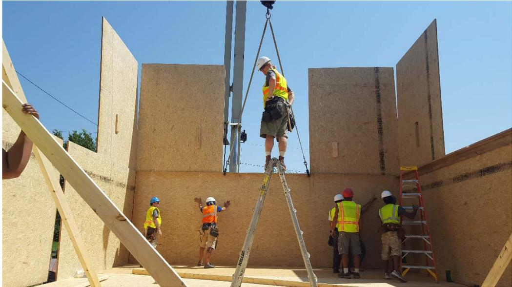
Figure B-6. Installing first floor interior horizontal panels
