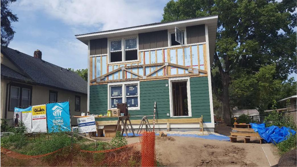
Figure B-17. Furring strips over foam for fiber-cement cladding installation (note porch connection)
