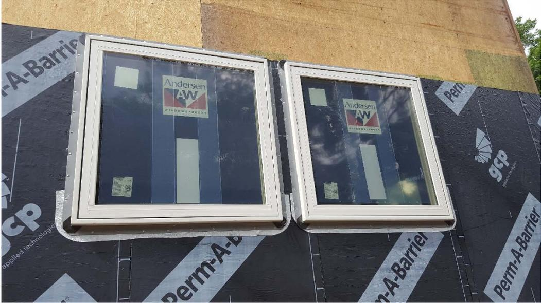
Figure B-15. Lower-level window installation integrated with air, water, and vapor control membrane
