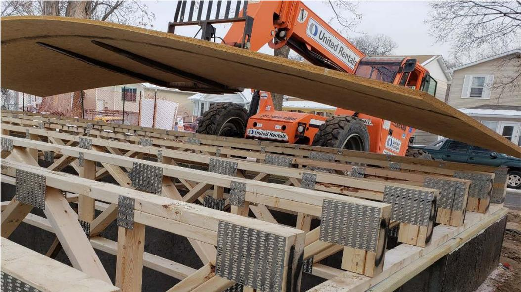
Figure B-4. First floor sheathing installation
