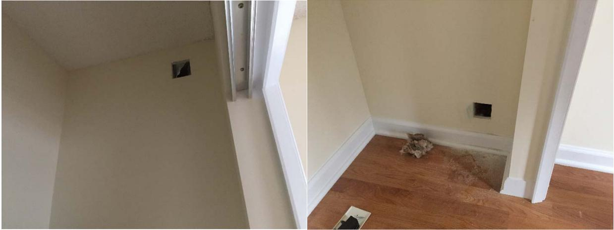
Figure 12. Typical moisture sensor installation in a frame wall showing top and bottom stud cavity locations
