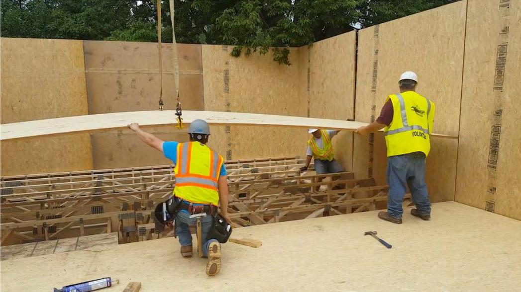
Figure B-7. Installation of second floor joists and sheathing
