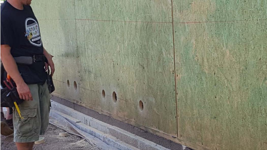
Figure B-13. All penetrations (with a couple of spares) are pre-located and cut
