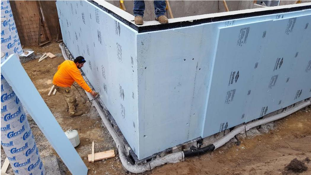
Figure B-1. Basement foundation with control layers
