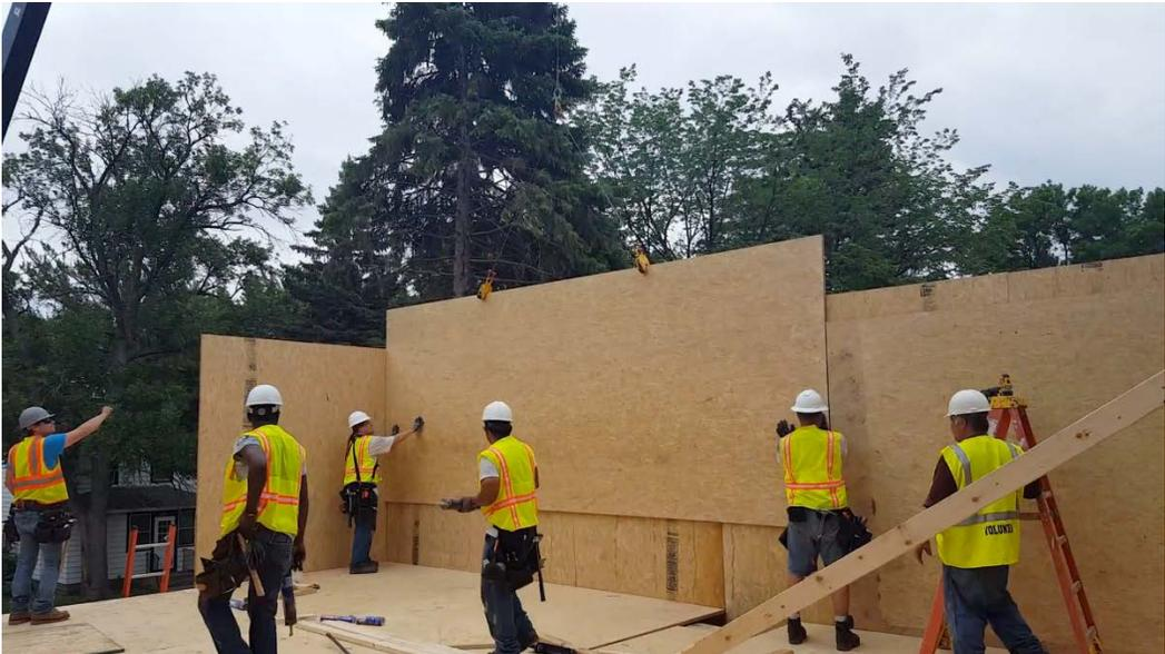
Figure B-8. Installation of second floor interior horizontal panels
