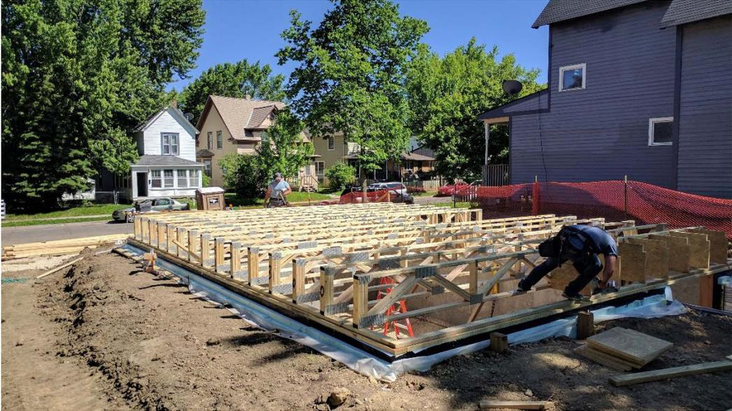
Figure B-3. Receiver plate and first floor joists installed
