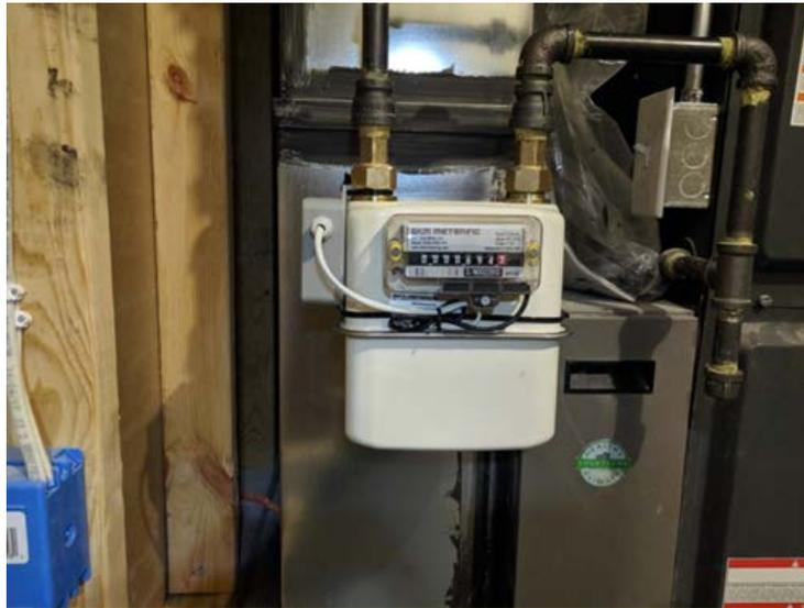
Figure 7. Typical natural gas submeter installation
