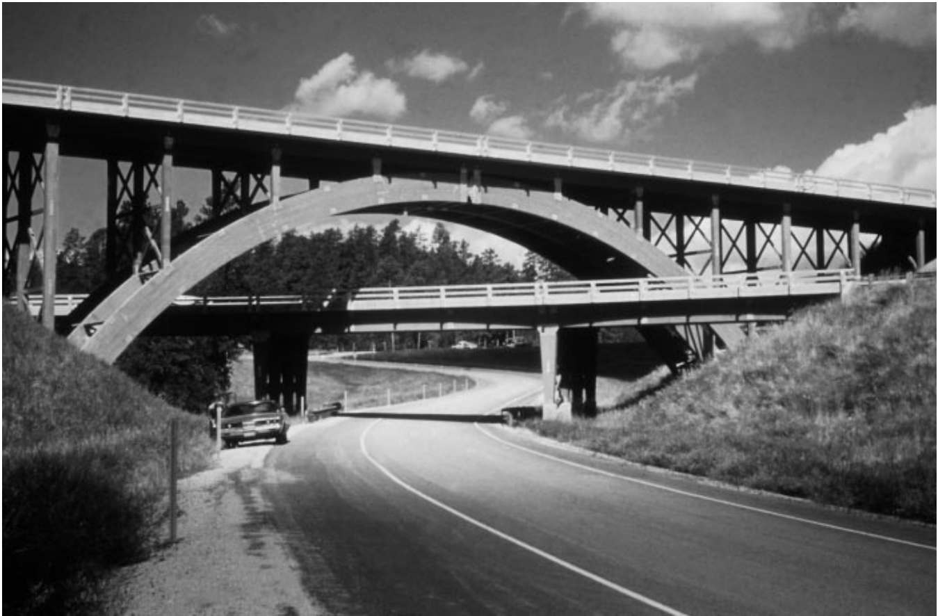
Figure 16–10. Three-hinge glulam deck arch bridge at the Keystone Wye interchange off U.S. Highway 16, near Mount Rushmore, South Dakota. The arch spans 47 m (155 ft) and supports an 8-m- (26-ft-) wide roadway.
