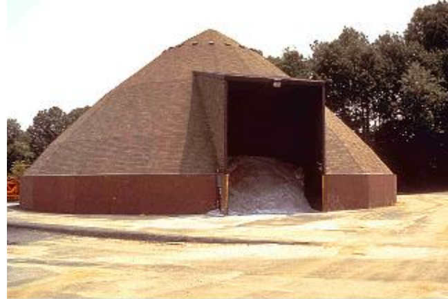
During storage, road salt should be covered to prevent salt from lumping together or being lost with storm water runoff
