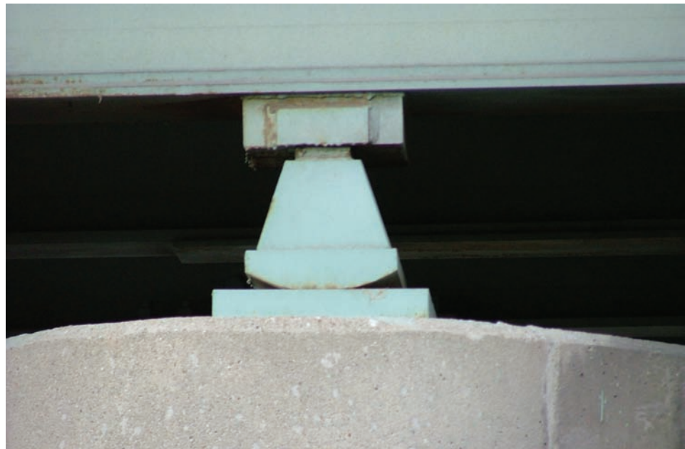
Figure 9.1.9 Rocker Bearing
