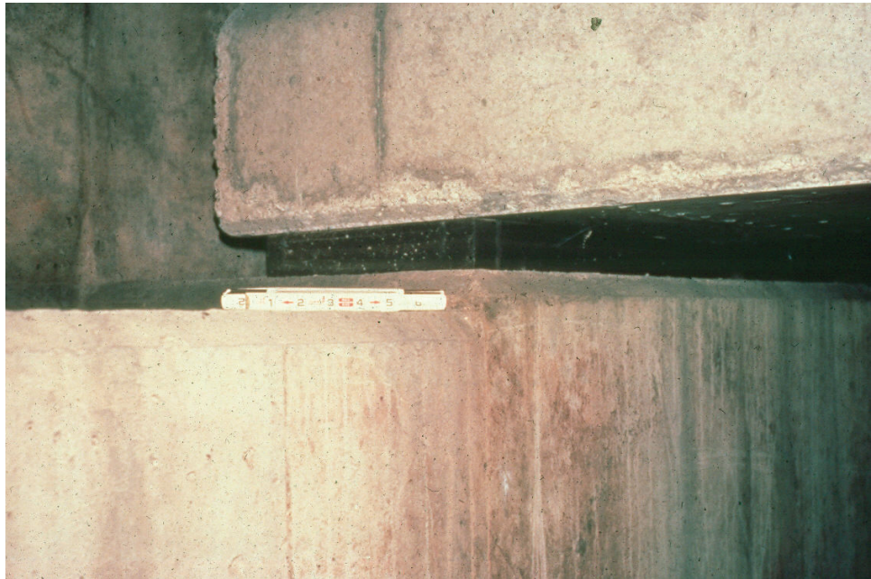
Figure 9.1.13 Plain Neoprene Bearing Pad
