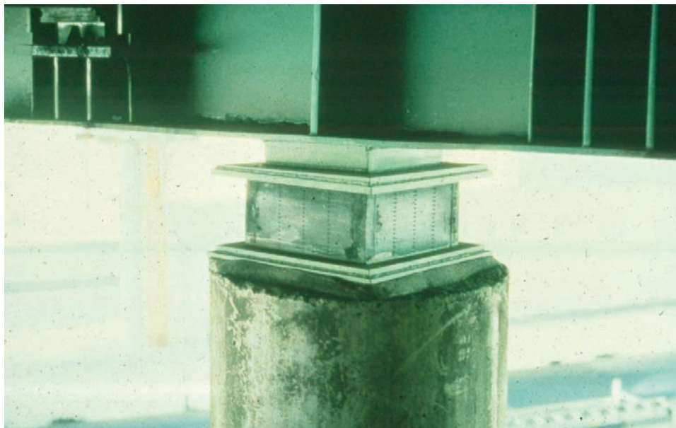
Figure 9.1.36 Lead Core Isolation Bearing
