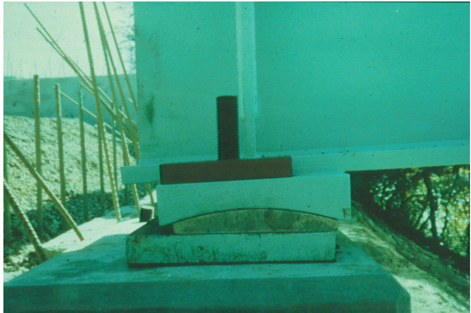
Figure 9.1.5 Bronze Sliding Plate Bearing
