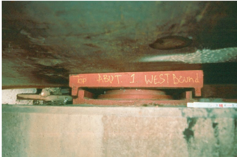
Figure 9.1.18 Pot Bearing
