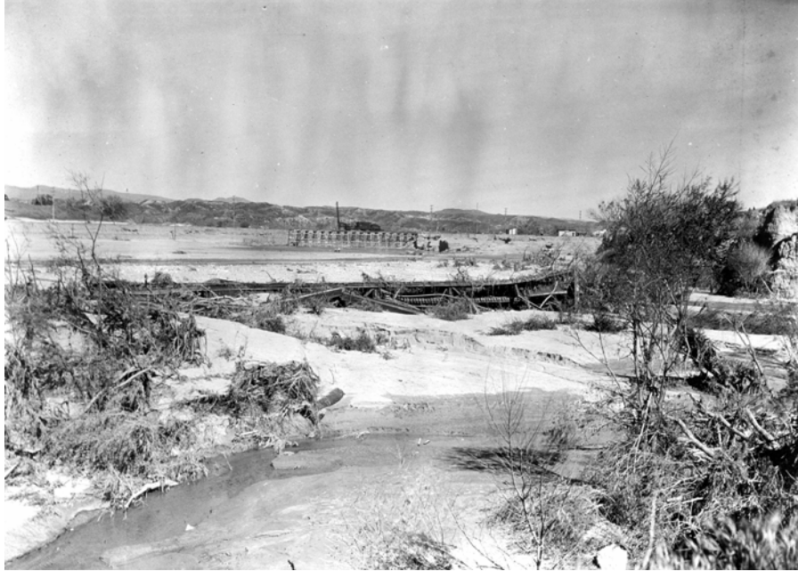
Highway damage (Attribution: U.S. Geological Survey Photographic Library) Figure 10
