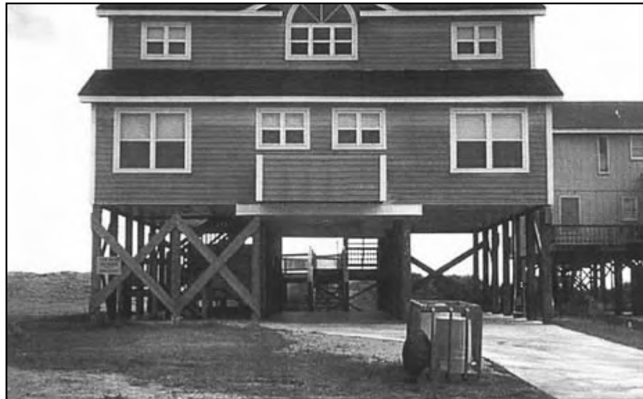
Figure 13-8 Diagonal wood bracing in a wood-pile foundation.
