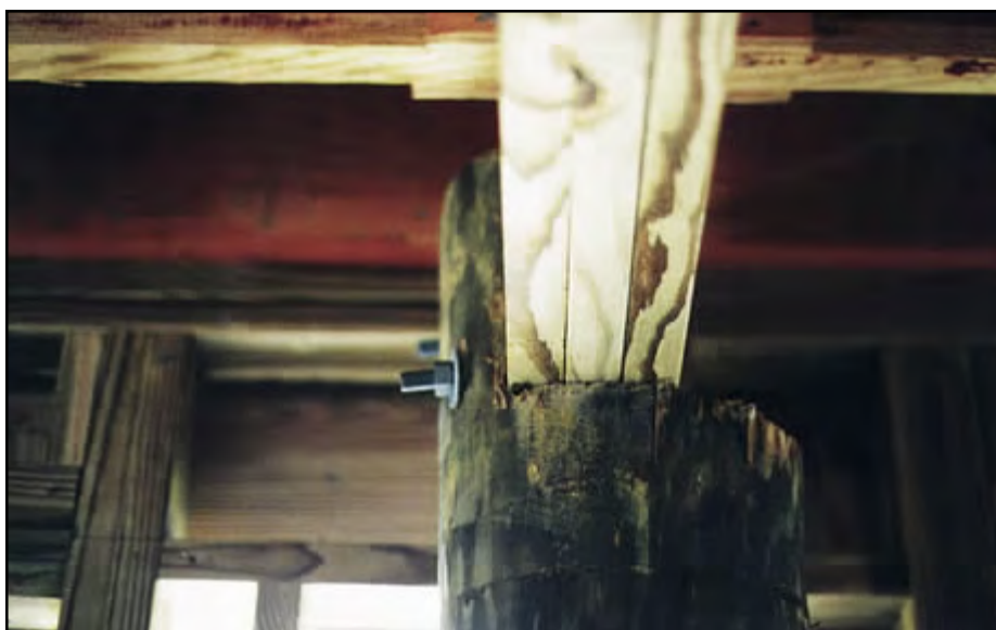
Figure 13-3 Overnotched pile. Also note mislocated bolt.
