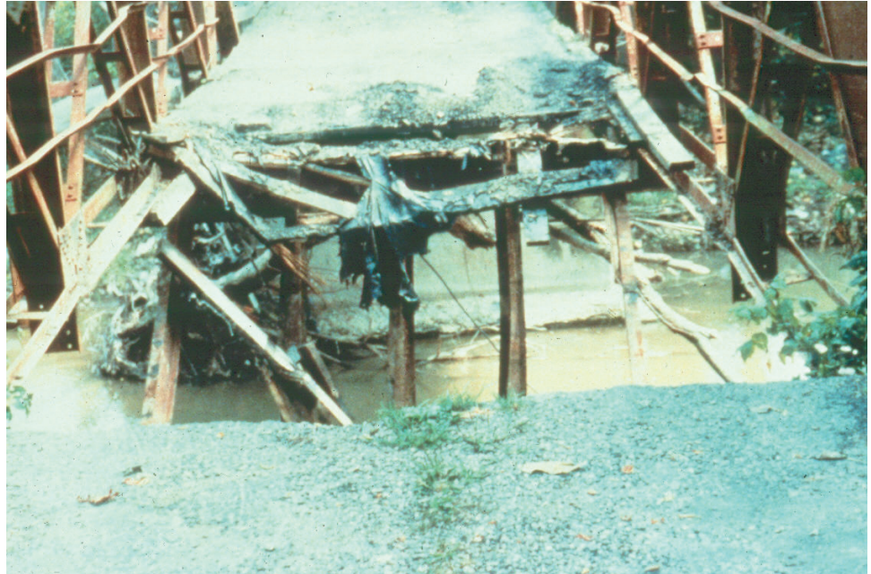
Figure P.2.21 Damaged Bridge due to Failure to Comply with Bridge Posting
