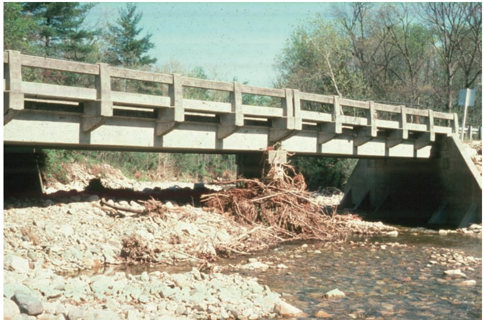
Figure P.2.27 Integral Bridge
