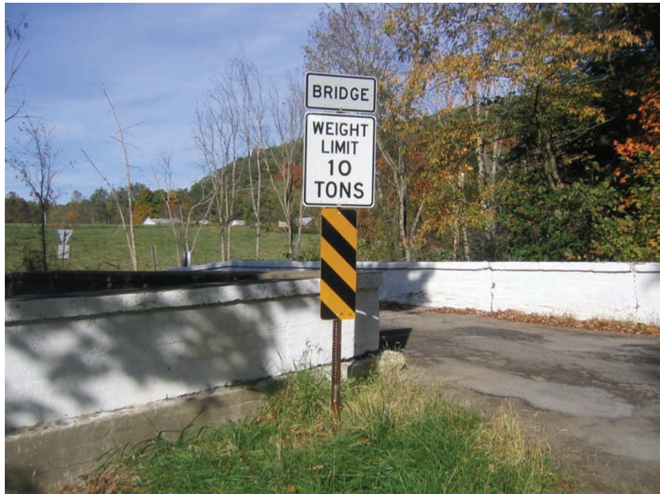
Figure P.2.20 Bridge Weight Limit Posting
