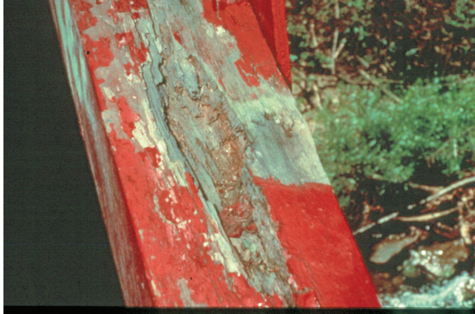
Figure 2.1.7 Decay of Wood by Fungi
