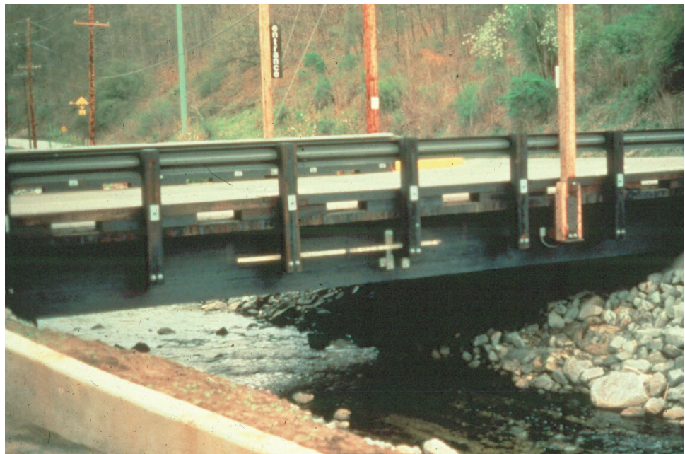
Figure 2.1.1 Glued-laminated Modern Timber Bridge
